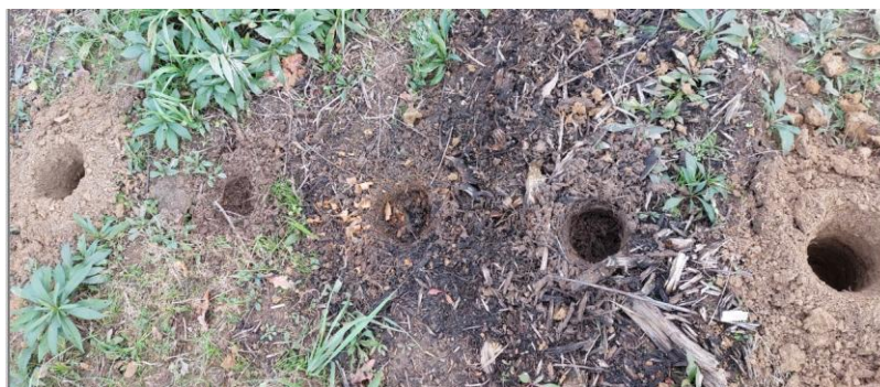
Figure 6: Drilled planting holes
