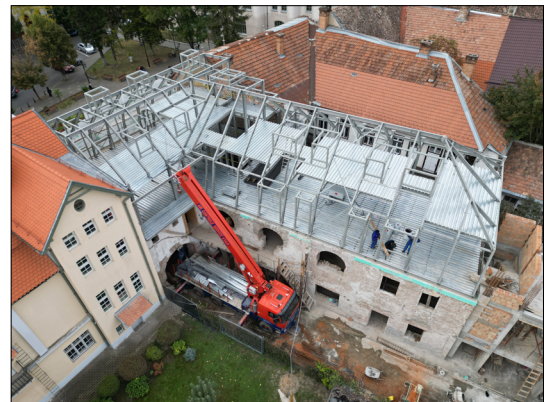
Fig. 3. Bolyai street 11 roof structure during construction.
