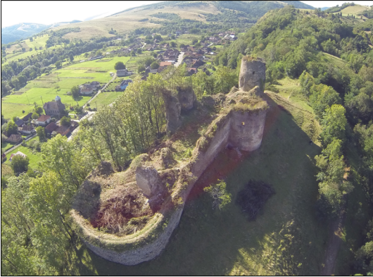
Fig. 5. Sebesvár castle before restoration.
