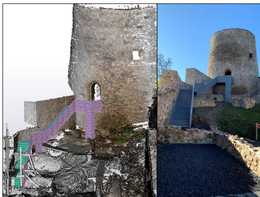
Fig. 4. Designed and executed staircase.
