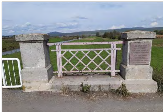
Fig. 2. The current state of the old bridgehead.
