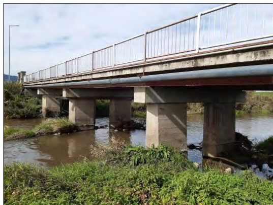
Fig. 9. Deposited riverbed sediment.
