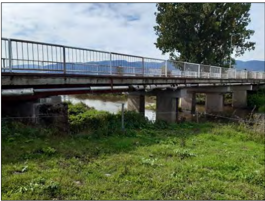
Fig. 4. The road bridge built over the widened riverbed on the site of the old arched bridge.
