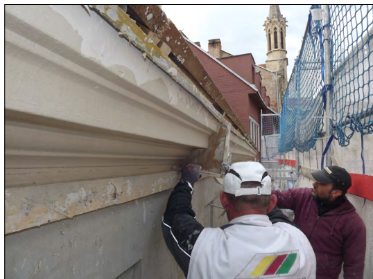
Figure 2. Moulding the fascia of the St. György street façade of 2 Hátsókapu, using a mould knife (author's photograph).
