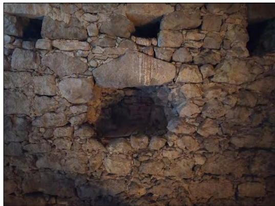
Figure 2. The three smaller holes and one bigger hole with a stone functioning as a lintel in the attic's gable wall.
