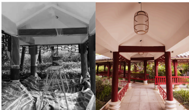
Fig. 2. Pavilion and corridor restoration (Source: Authors)
