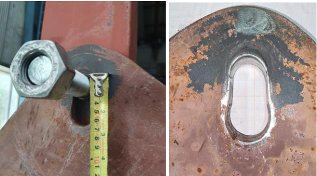
Figure 6 Failure mode obtained in the tests.
