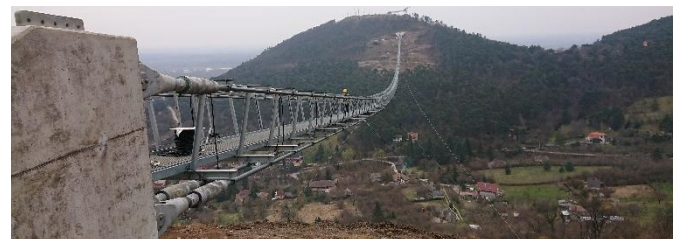
Figure 1 View of the bridge
