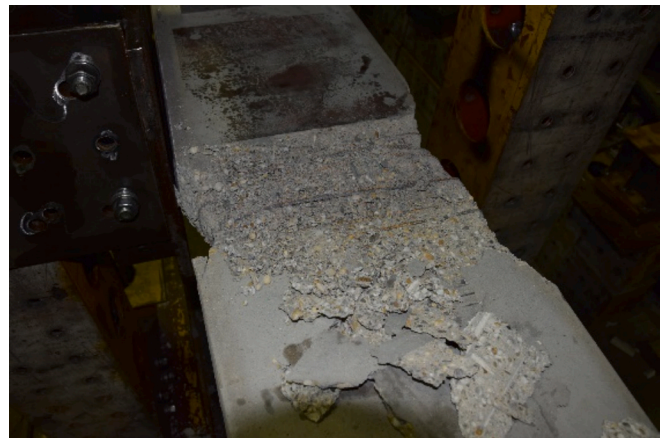
Fig. 23. Upper concrete flange failure (B3) – view from above.
