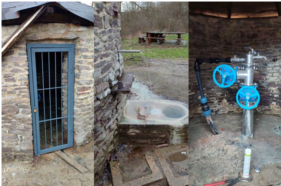
Photo 2. Closure of the well site Photo 3. Groundwater discharge from the overflow Photo 4. Reconstruction of the TMS-2 borehole wellhead
