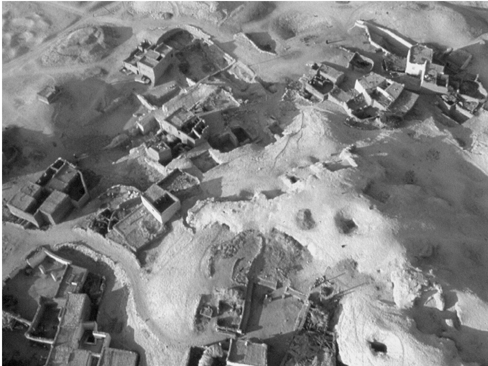
Fig. 2. The south slope of El-Khokha from the air, taken before the beginning of the excavation (1995). In the centre of the picture, in front (left) of the rock line of the façades of the New Kingdom tombs in the uppermost section of the hillock there is still no sign of any structure. (Photo: György Csáki)
