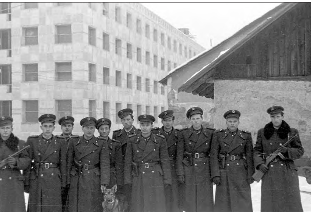
Police at construction site in Salgótarján, 1952
