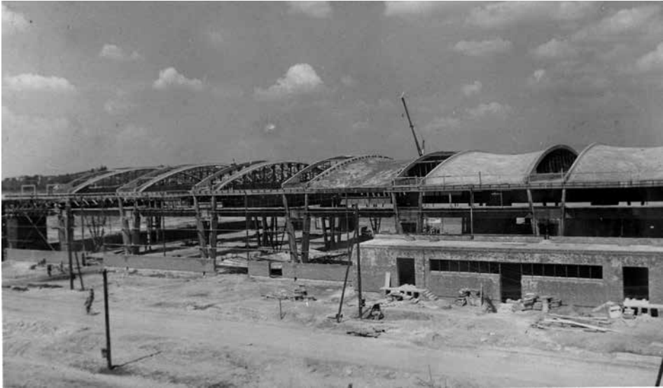
Figure 9. KÖFÉM factory during construction
