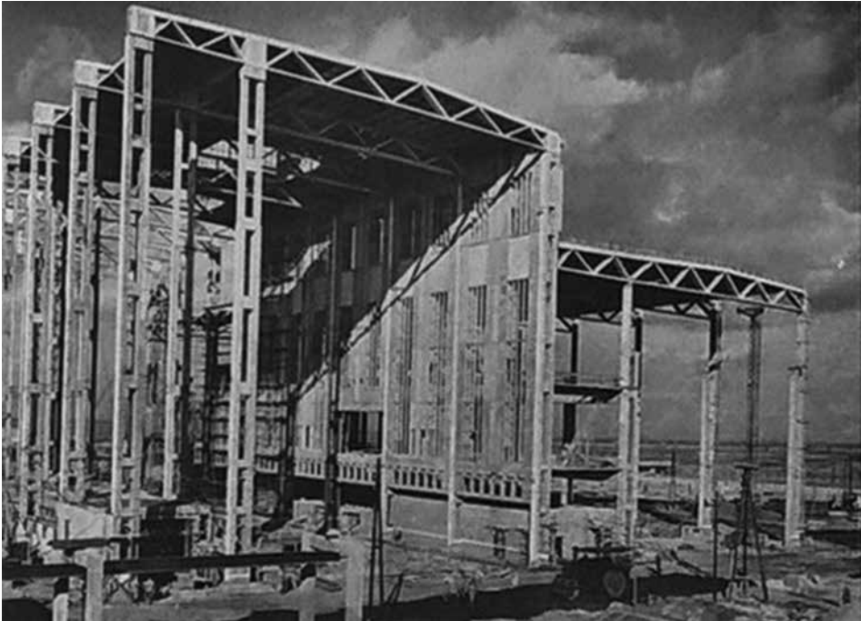
Figure 1. Thermal Power Station, Tiszaújváros (H) (Mátrai, Pászti, 1955) an example of the industrial buildings erected in the early fifties, using reinforced concrete and large-scale-on-site-prefabrication technic
