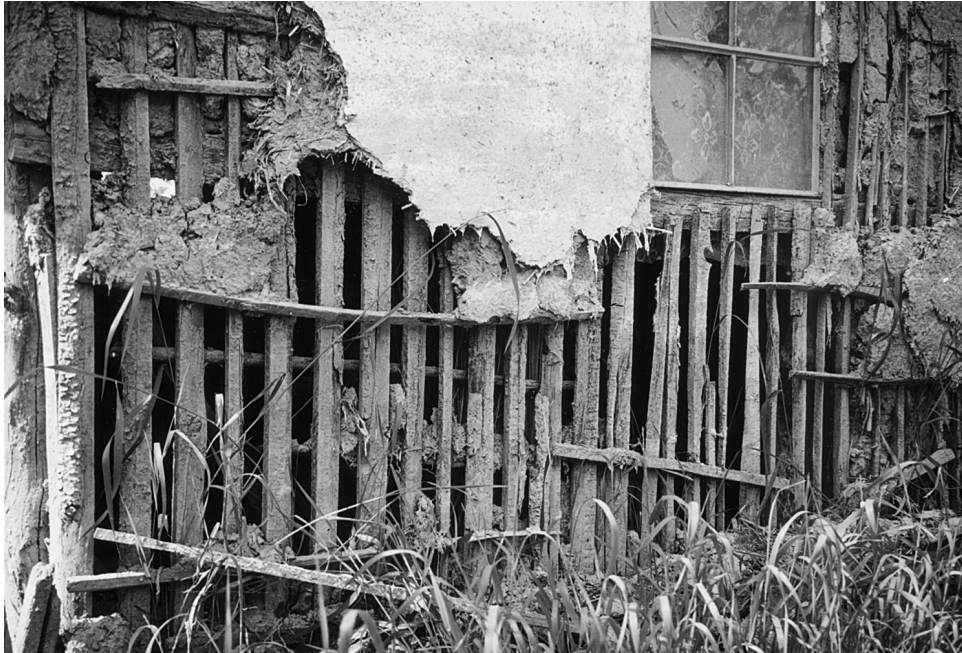
Fig. 1. Light timber frame wall structure (Szentcs, 1999)
